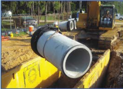
Steel Trench Shield
