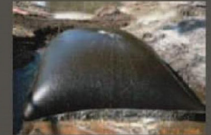
Dewatering Bags for containment of filtered sediment
