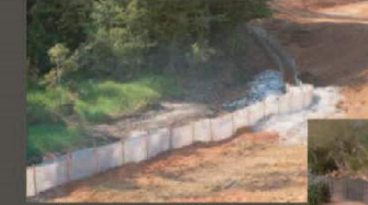
Wire-backed & Scrim Reinforced Silt Fence for site-specific applications
