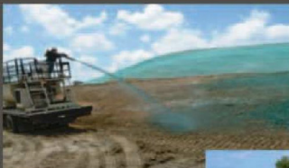
Hydroseeding Mulches & Additives for temporary erosion control & permanent turf establishment
