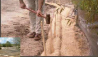
Rolled Straw & Wattles as silt fence alternative, perimeter & sediment filtration on slopes
