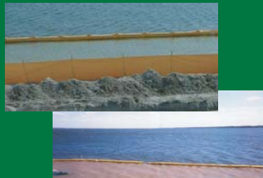
Floating & Staked Turbidity Barrier for controlling sediment transport in waterways, streams & creeks
