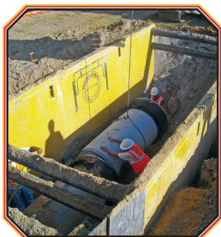
steel trench shield
