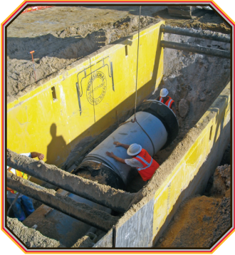
steel trench shield
