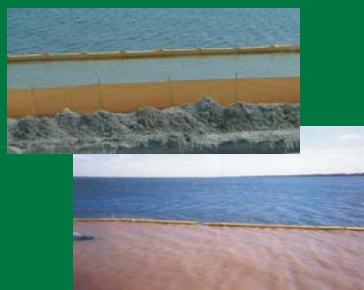
Floating & Staked Turbidity Barrier for controlling sediment transport in waterways, streams & creeks
