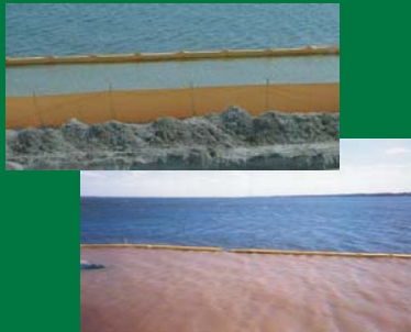
Floating & Staked Turbidity Barrier for controlling sediment transport in waterways, streams & creeks
