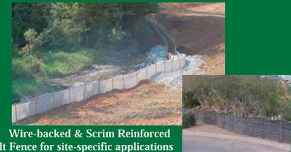
**Wire-backed & Scrim Reinforced Silt Fence for site-specific applications**
