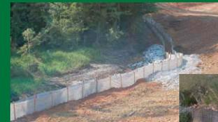
**Wire-backed & Scrim Reinforced Silt Fence for site-specific applications**
