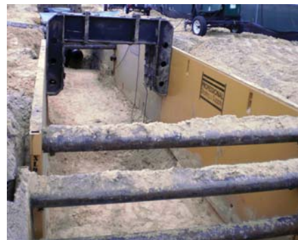
The trench shields (also known as trench boxes) were 8' tall, 24' long XLD Series shields with 4 inch sidewalls manufactured by Efficiency Production, Inc. and provided by Professional Shoring & Supply.
