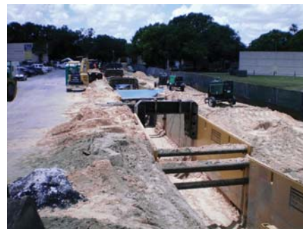
To facilitate the protection of workers installing and welding the pipes in the trench excavation, Dallas 1 employed a series of trench shields to shore the pipeline.
