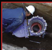
Occlude isolation valve bolted in place
