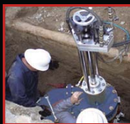
Tapping machine installed
