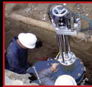
Tapping machine installed
