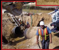
36" Line Stop and Pipe Cutting
