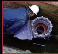
Occlude isolation valve bolted in place
