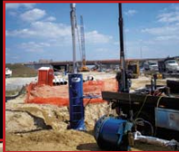
36" Line Stop and Pipe Cutting
