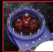
Bonnet & Gate installed in valve body, insert tool removed
