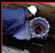
Occlude isolation valve bolted in place
