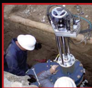
Tapping machine installed
