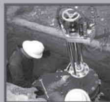
Tapping machine installed
