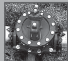
InsertValve™ with bonnet ring bolted in place, install complete.
