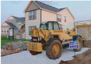
RESIDENTIAL CONSTRUCTION ENTRANCE
