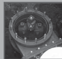
Bonnet & Gate installed in valve body, insert tool removed
