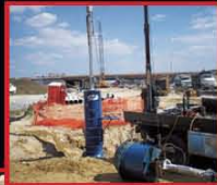
36" Line Stop and Pipe Cutting
